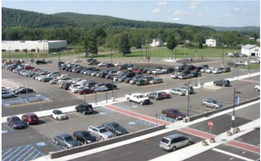
ELM's completed parking lot and entrance drive
