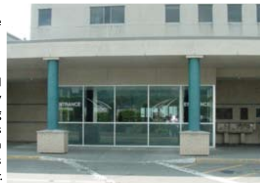
New Airport entrance featuring new doors and carpeting have replaced a non-functional revolving door.
