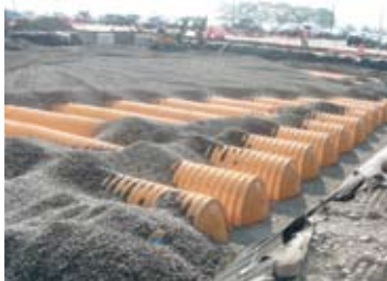
Counterclockwise from left: underground stormwater detention system in place; excavation work underway; FAA cable installed. Every area in these photos will be paved over and become NEW parking.
